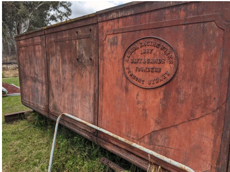
View of northern elevation of the derelict Water Tank illustrating a broken panel with builder's mark.
