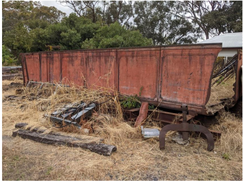
View of western elevation of the derelict Water Tank illustrating a broken and collapsed corner panel.
