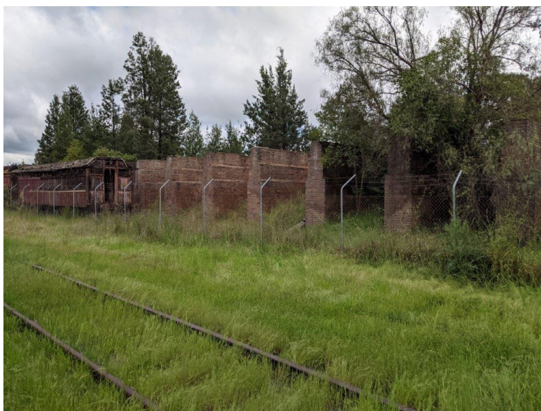
View of the eastern elevation of the Elevated Coal Bunker and De-ashing Plant illustrating remnant brick piers.
