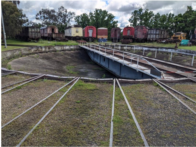
View looking east at the Turntable, with Turntable Roads in foreground and “bull ring” roads in background (all part of element 29), illustrating rolling stock stored on the latter.
